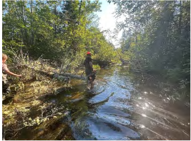
Section of Belle River after clearing
