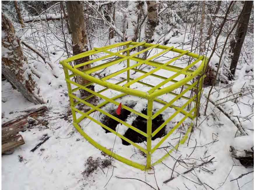
In progress installation of protective cage at bat monitoring station
